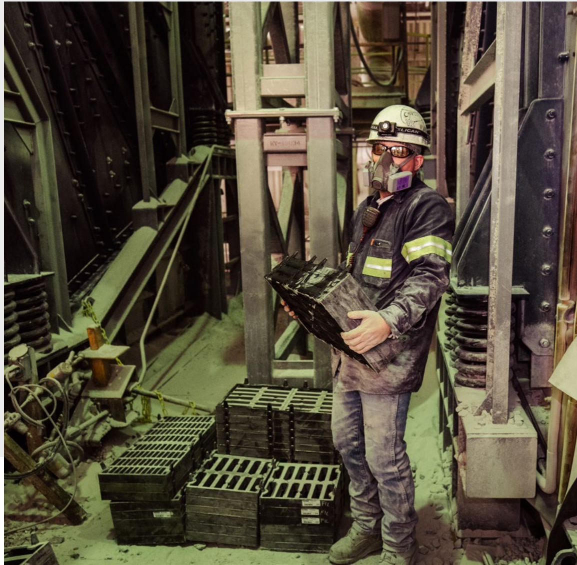
*Image shows Pinto Valley employee during a block changeout, replacing Rubberdex XLR® panels.
